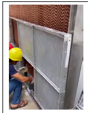
Air Filters Installation
